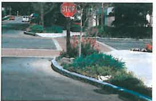
Corner bump-outs, landscaping and pavement, and stop sign as ways to calm traffic.
