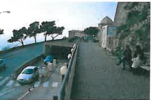
A buried parking garage under a park.
